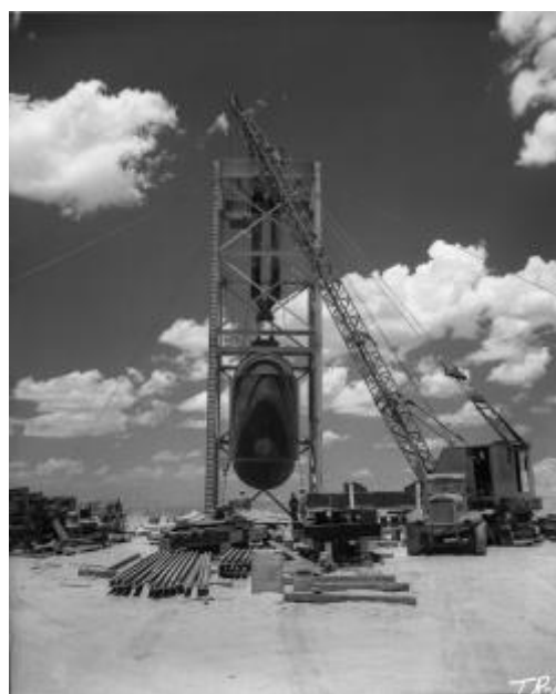
Image 2 - 1st Nuclear Device Test - Operation
